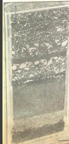
Core section of track surface Trinidad tar is first layer
